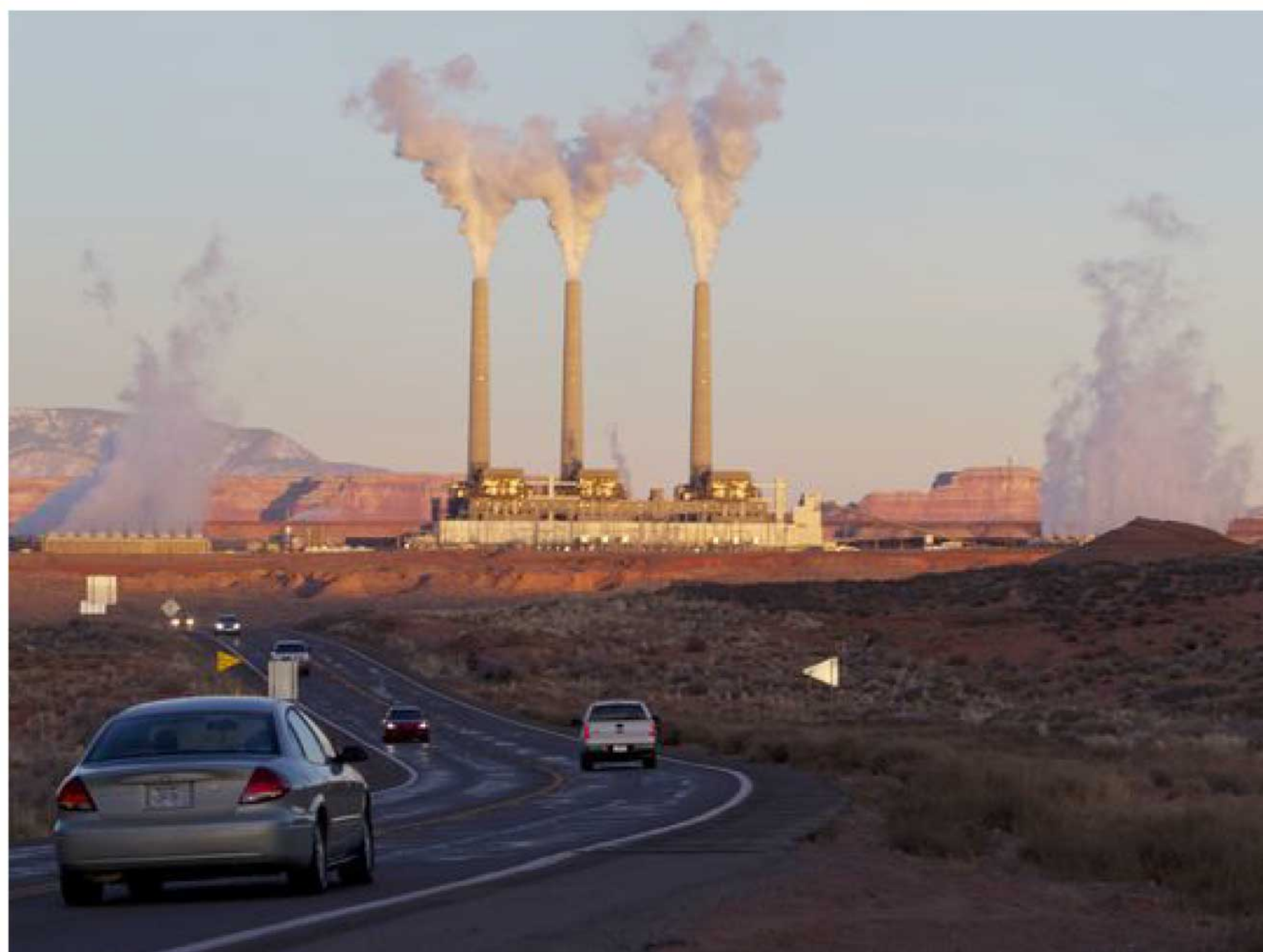
Evaporated water leaves the tops of stacks at the Navajo Generating Station near Page. (Photo: Patrick Breen/The Republic)
